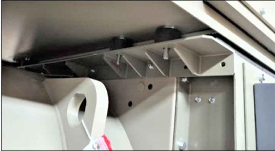
FIGURE 12. WATER COOLER LOWERED IN TO POSITION
